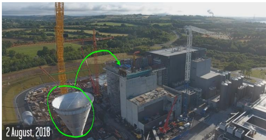
Figure 7: Drier Unit Installation at a Glanbia Facility under Construction.
